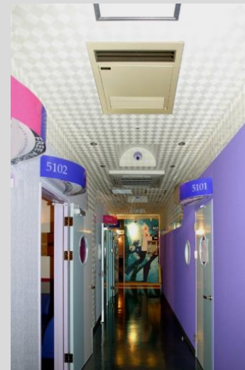
Ceiling-installed cassette type PTC Steam Humidifier TJ2000T Series
